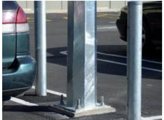
Cast in bollards to protect light poles in carparks.
