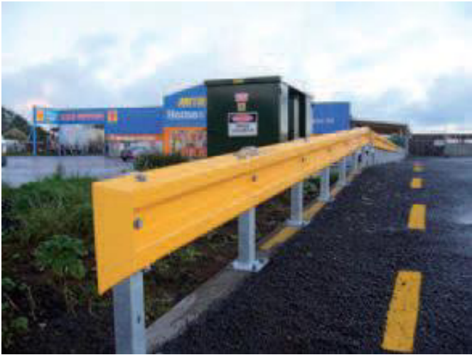
Protect transformers from traffic.
