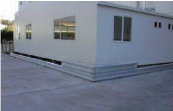
Two high barrier to protect the corner of a building from traffic damage.
