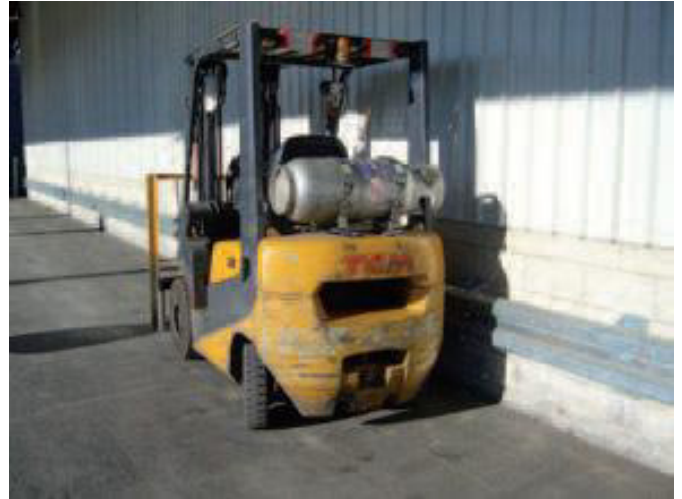
Galvanised barrier bolted to the wall to stop fork damage to the wall and cladding."
