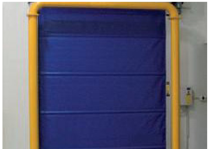
Full frame bollard to protect the rapid acting door.
