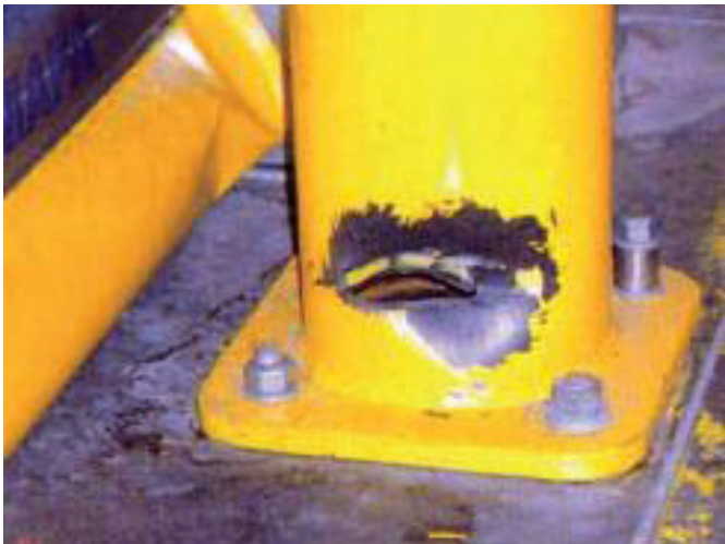
A standard bolt down bollard with a fork hole in. Admittedly hit in the strongest place, but it was there to protect the door from the next forktruck.
