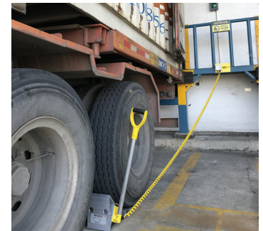
Coil cord communicates between wheel chock and Dok-Lok Style Light Communication System
