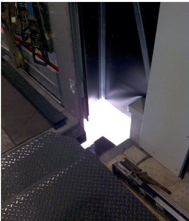
Exposed bottom corner gaps equal up to a 0.50 m 2 opening allowing contaminants to enter the facility and expensive energy to escape.
