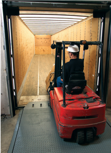
Ordinary (collapsible) dock shelter leaves trailer door hinge gaps exposed.
