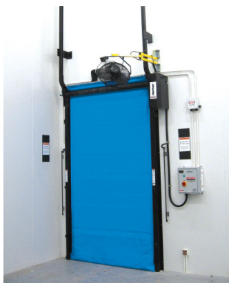
Vertical Lift - A vertical lift routes the FasTrax tight to the wall, when there is ample ceiling height.
