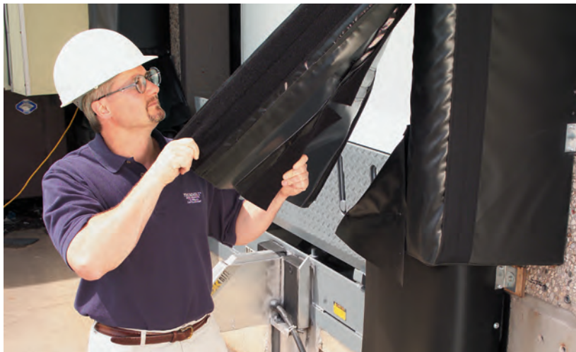
Removable side curtains allow for maintenance flexibility.
