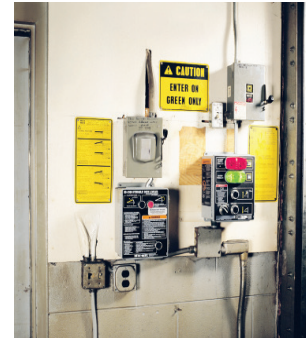
Multiple controls at each dock position can be complicated and potentially dangerous
