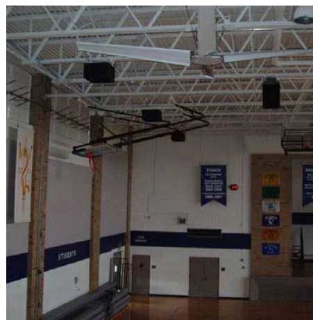
Gymnasiums and Field Houses
